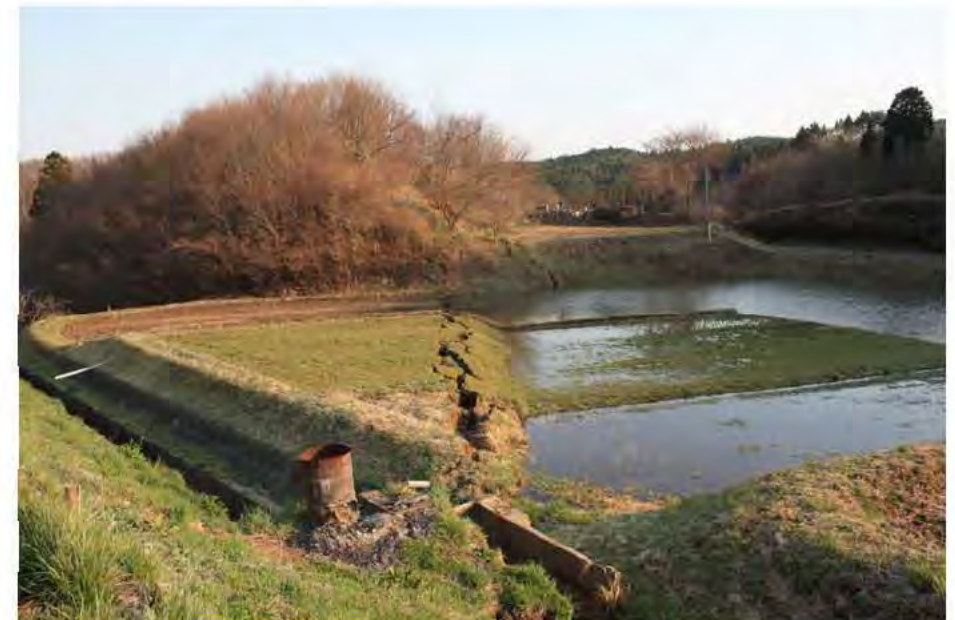
Surface rupture associated with the 2011 Hamadori earthquake (M7.0).4.11
