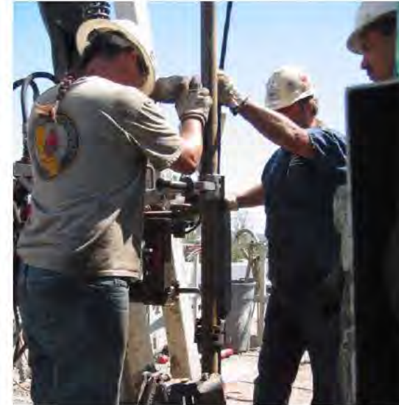
Pilot Hole VSP Array – Installed on 2 3/8" Production Tubing
