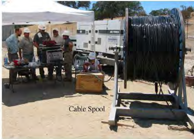
Pilot Hole VSP Array 32 Level 3-Component 15 Hz install between 800 to 2,100 m
