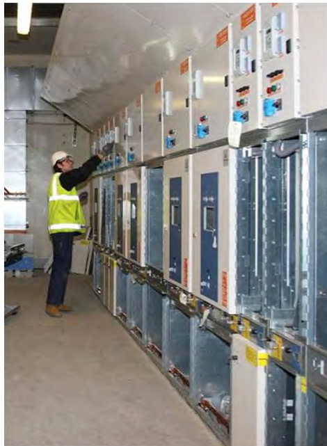
FA3 Electrical cabinets in installation
