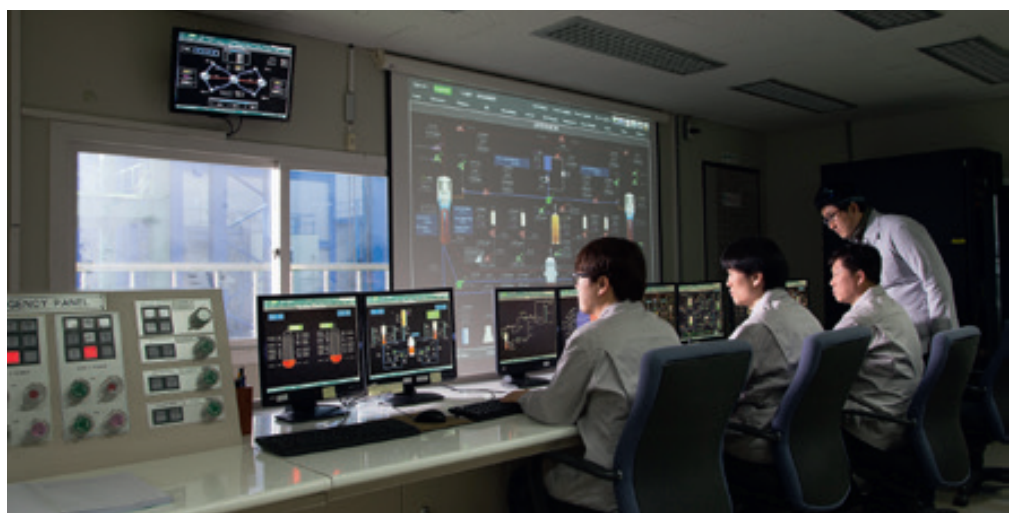
The ATLAS facility. KAERI, Korea
