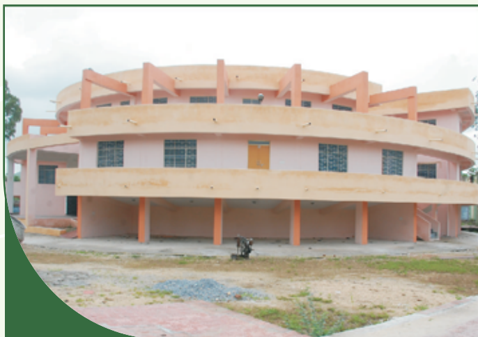
Students Instructional Block at CTAE : Four lecture theaters of 100 seating capacity two labs and equipped with modern teaching aids. The units of Basic Sciences, Environmental studies and English are housed in this block
