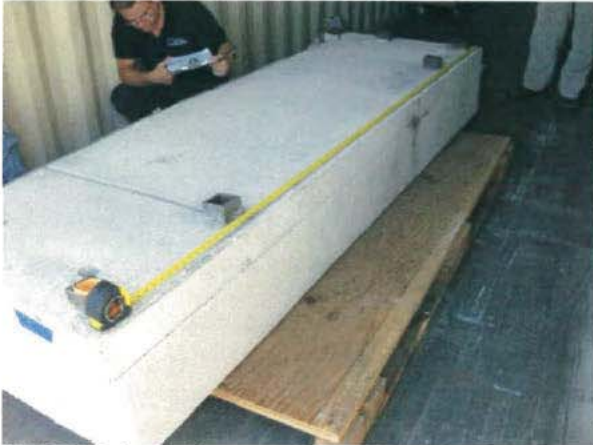
Unit 305 Balcony Remnants Photo 5667 – 29 July 2015
