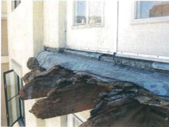
Unit 405 Balcony Photo 5458 – 29 July 2015
