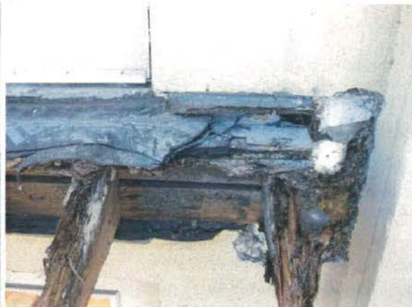
Unit 405 Balcony Photo 5459 – 29 July 2015
