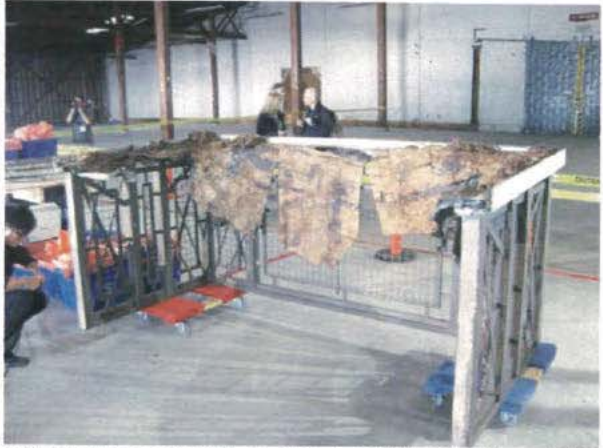
Unit 405 Balcony Remnant Photo 5978 – 6 October 2015
