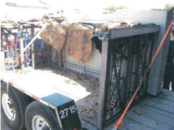
Unit 405 Balcony Remnants Photo 5498 – 29 July 2015
