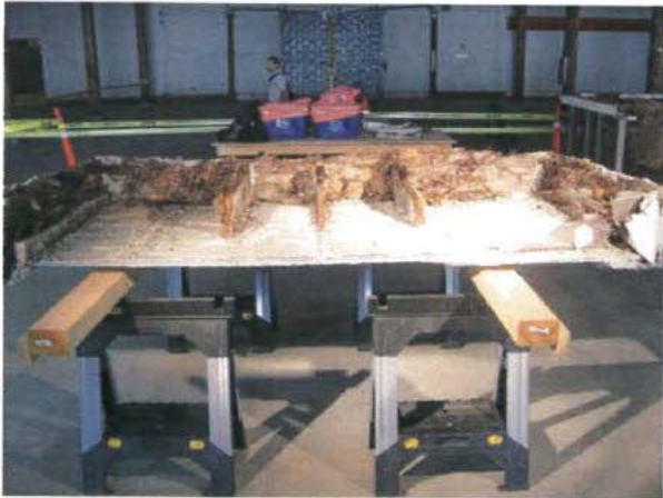
Unit 405 Balcony Remnant Photo 5954 – 6 October 2015
