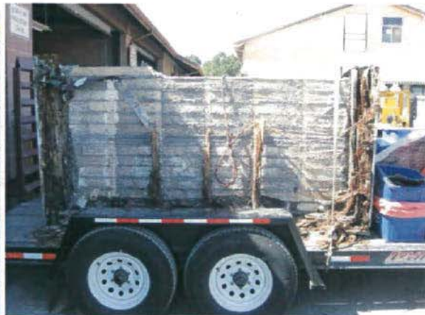
Unit 405 Balcony Remnants Photo 5616 – 29 July 2015
